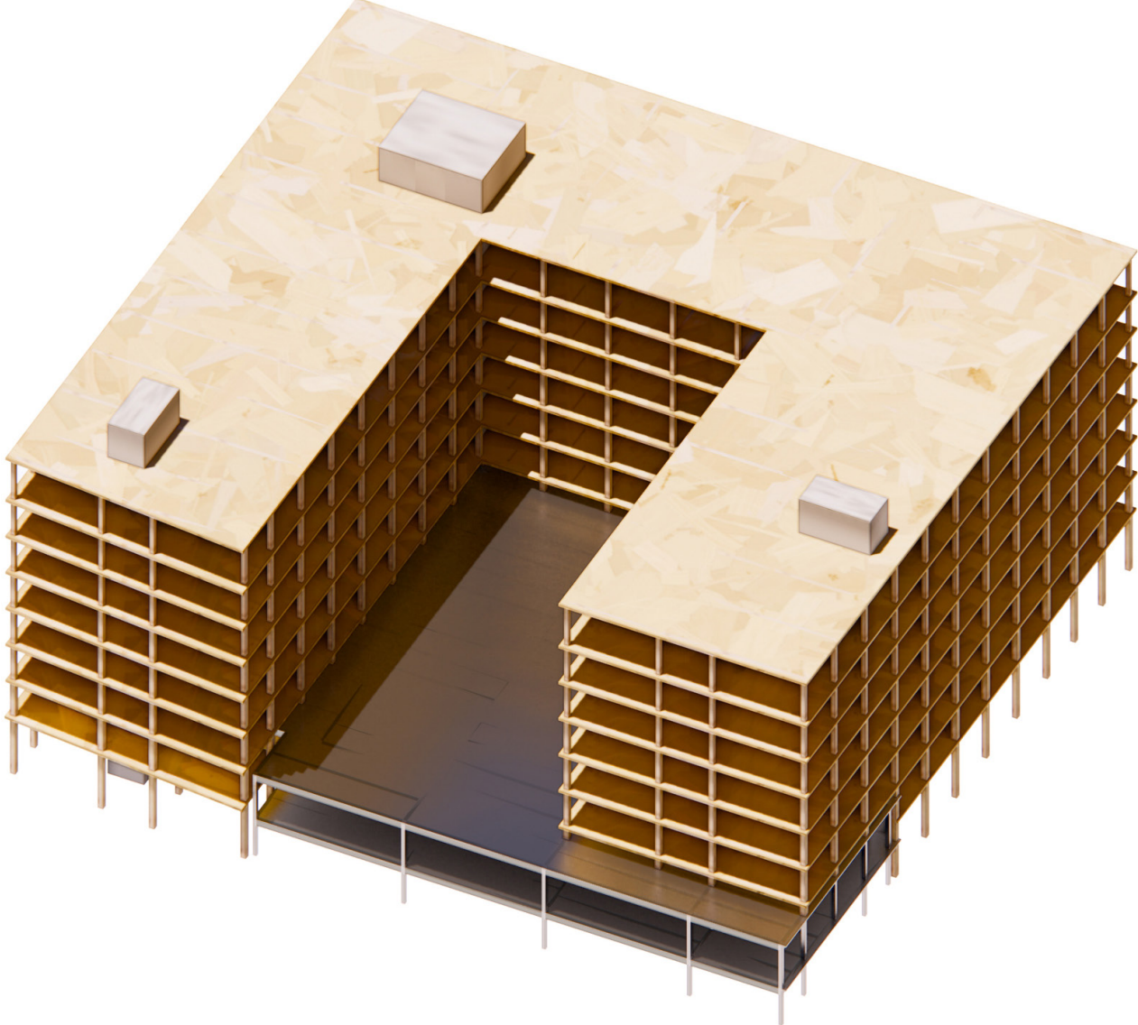
MASS TIMBER STRUCTURE
