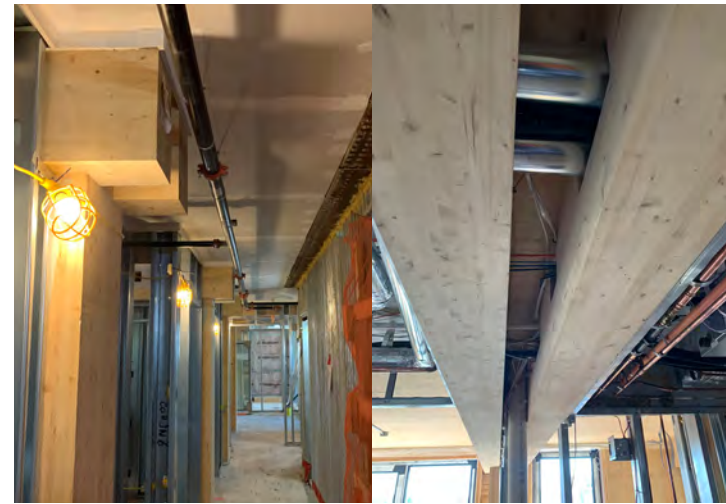
11 E Lenox corridor and beam penetrations precedent
