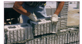
Fig. 1. Use a workable, water-retentive mortar. (MGT13629)
