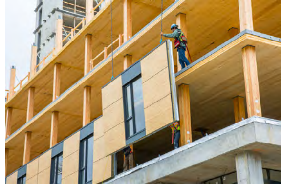
Architect: Acton Ostrey Architects Inc Photo credit: KK Law / Naturally Wood
