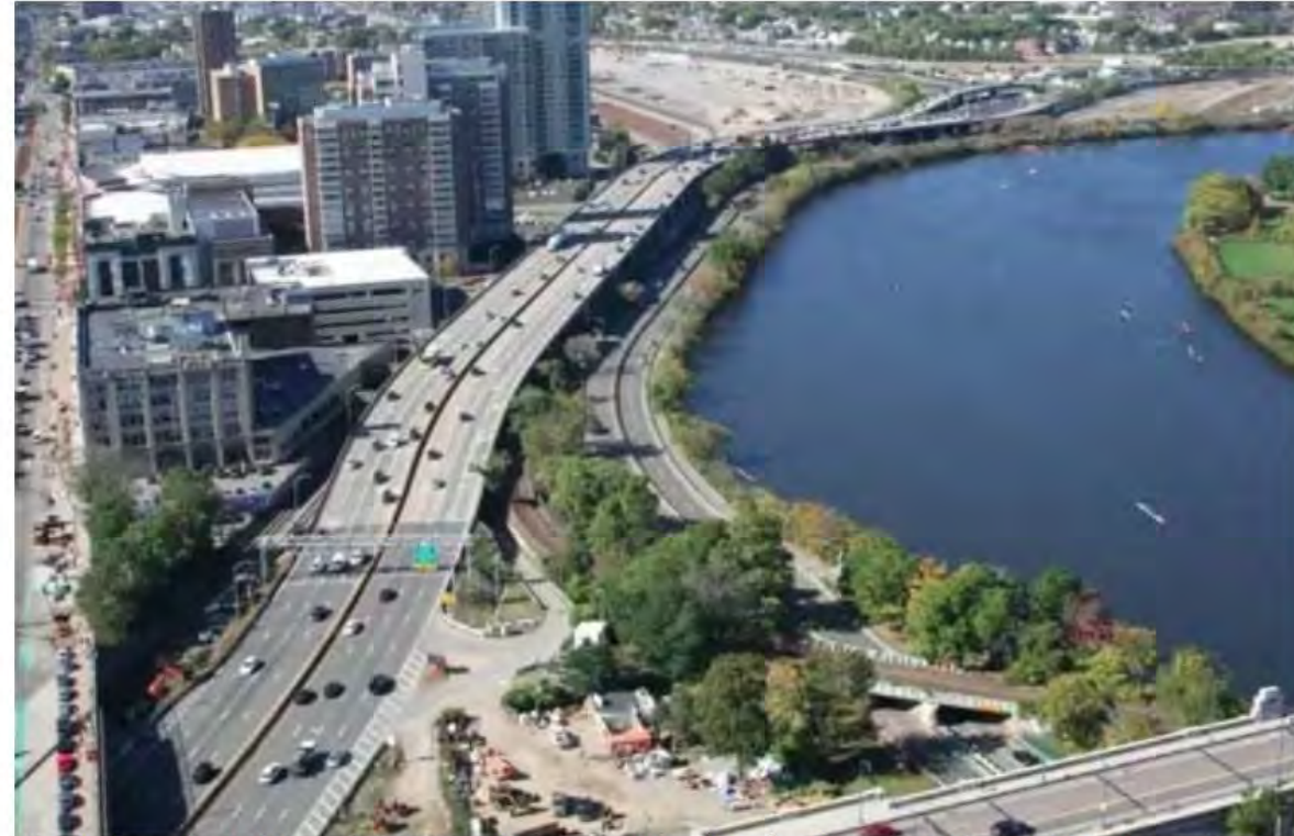
Picture shows elevated Massachusetts Turnpike between BU and Charles River with Soldiers Field Road at grade. The bend in the Turnpike at the top of the picture would be straightened if the broader project I-90 Allston interchange project is pursued.
