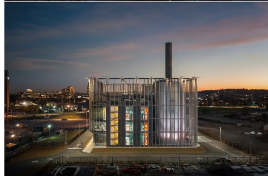
Images top to bottom: Metropolitan Area Outer Underground Discharge Channel Rose Fitzgerald Kennedy Greenway, City of Boston Central Signal Box, Herzog & de Meuron District Energy Facility, Leers Weinsapfel Associates
