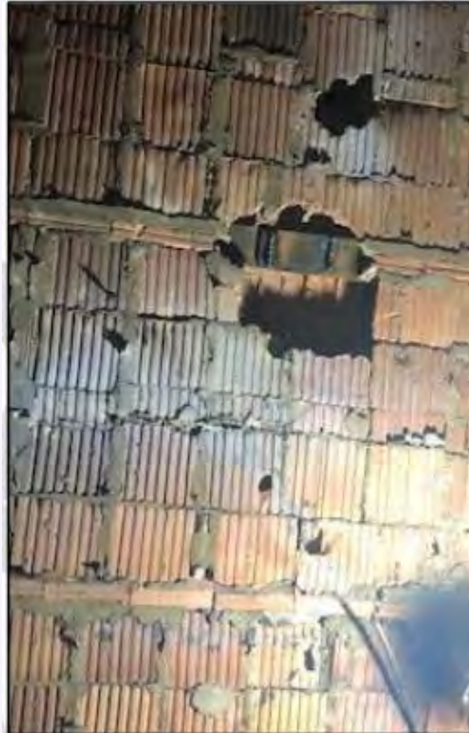
Figure 1: Photos of Damage to Condition Passive Fire Resistance Features
