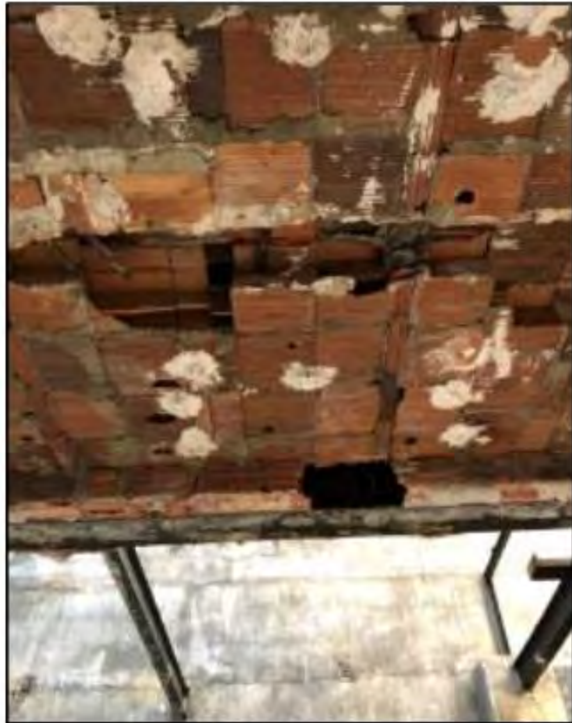
Figure 1: Photos of Damage to Condition Passive Fire Resistance Features
